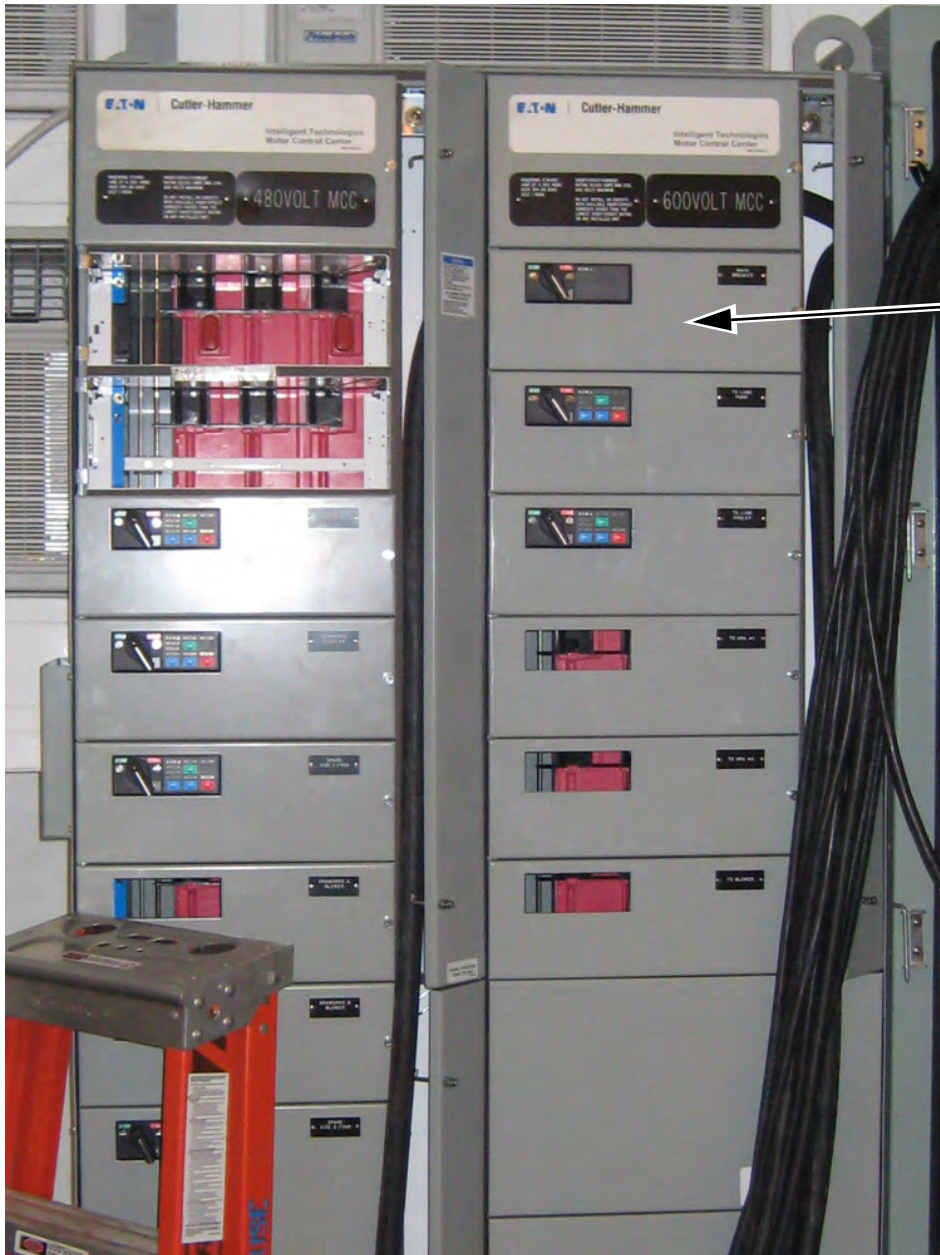
Figure 1: MCC Feeder Breaker for 600V section
